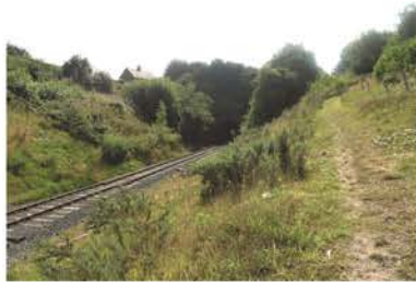
Above - Railway tunnel entrance from the Lawley Common side
